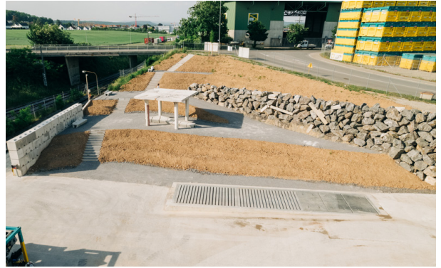
FIGURE 2. Aerial view of the retaining wall at Circularity Park. (© Gramazio Kohler Research, ETH Zurich, Eberhard AG. Photo: Marc Schneider)
